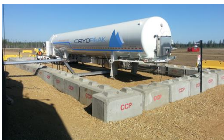
Figure 2.37, 2.38 and 2.39 – Two on the top representing fixed LNG bunkering installations, both with 3 horizontal pressure tanks. The one below representing an LNG trailer installed temporarily, with concrete defences and
