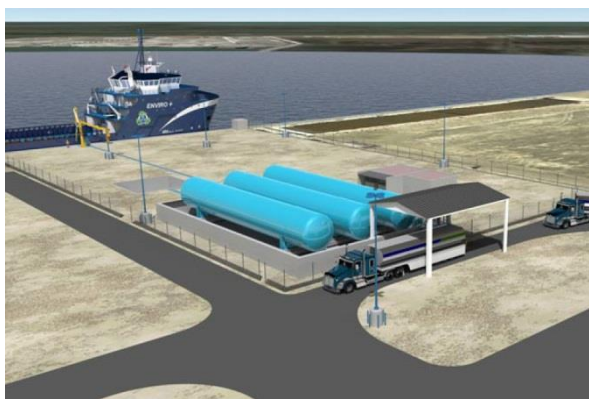
Figure 12.7 – Port-to-Ship (PTS) Bunkering. LNG bunkering fixed installation fed by LNG fuel trucks. This is, in practice, an alternative to improve the LNG delivery rate and volumes to the receiving ship. The fixed installation works here as a buffer station.
