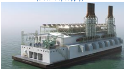
Figure 4.10 – LNG fuelled floating power plant
