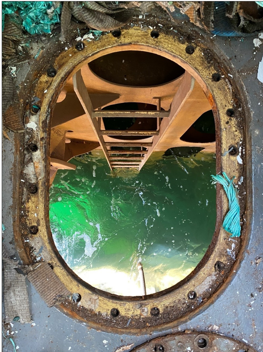
Photo credit by BSU (Germany)
